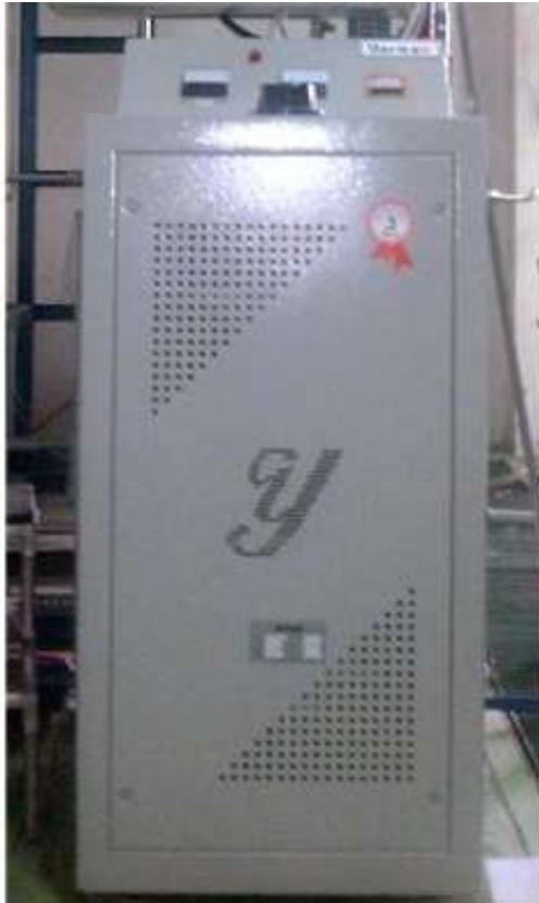
Gambar 5. Slide regulator voltage.
